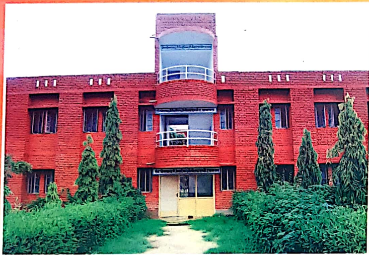
Well Equipped Boys Hostel
